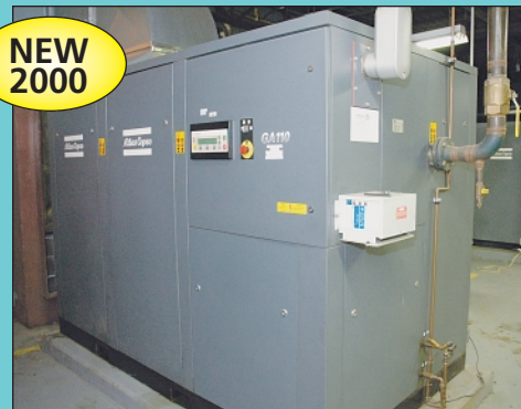
NEW 2000 150 HP Atlas Copco Model GA110 Cabinet Enclosed Rotary Screw Air Compressor
