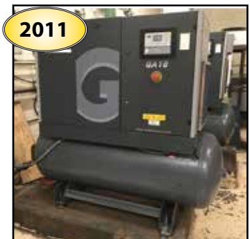
(3) ATLAS COPCO GA 18 Air Compressors
