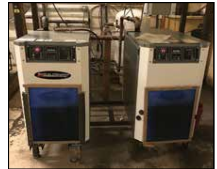
(2) AIRTEK Infiltration Air Treatment Packages
