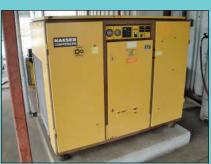
40 HP Kaeser Model BS-50 Rotary Screw Cabinet Enclosed Air Compressor
