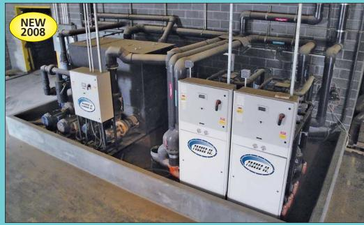
(2) Freeze Model FCCWC-0050 Compact Water Cooled Central Chiller Systems and Freeze Model PNL-130 Insulated Chilled Water Tank
