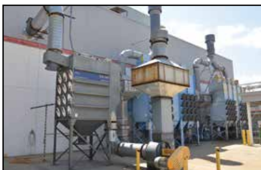
SULZER METCO SMEOVAL-36 Dust Collector
