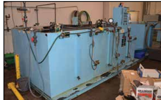
MASTER CHEMICAL Coolant Filtration System
