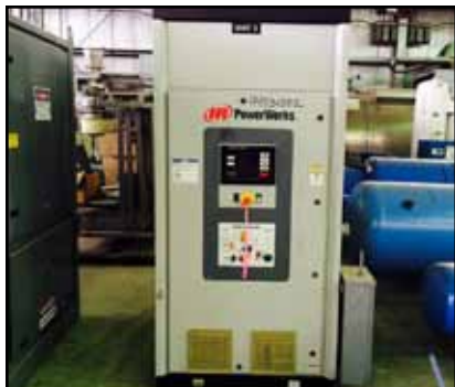
INGERSOLL-RAND PowerWorks 70 kW Microturbine / Peak Shaving Natural Gas Generator Set
