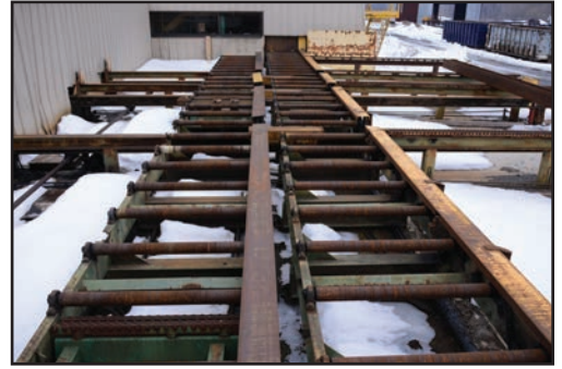
(2) 56' X 43" POWER ROLLER EXIT CONVEYORS
