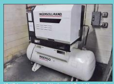
15 HP Ingersoll Rand Horizontal Tank Mounted Air Compressor
