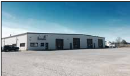
817 Progress Drive – 6.767 acres w/14,500 SF commercial building
