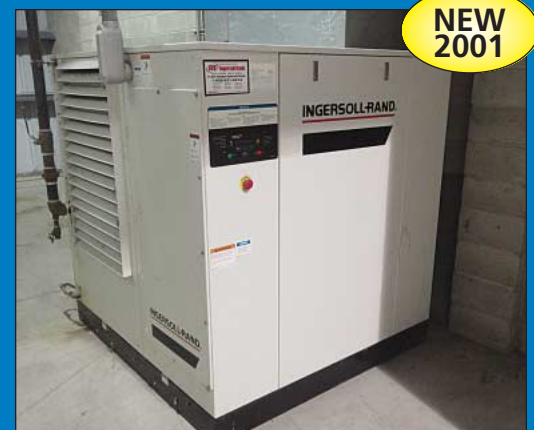
100 HP Ingersoll Rand Model SSREP-100 Rotary Screw Air Cooled Air Compressor
