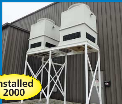
(2) AEC Model FG-2003 Fiberglass Cooling Towers
