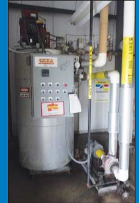
Geka Type THZ4.40 Propane Gas Fired Hot Oil Heater
