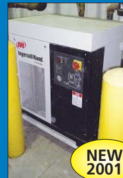
Ingersoll Rand Model TS500 Refrigerated Compressed Air Dryer
