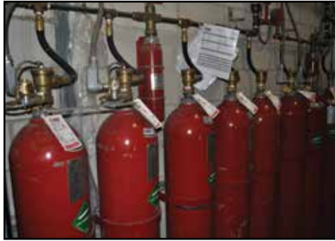
FIKE SHP-Pro CO2 Fire Suppression System
