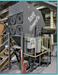
Torit Model DFT2-8 Cartridge Type Dust Collector
