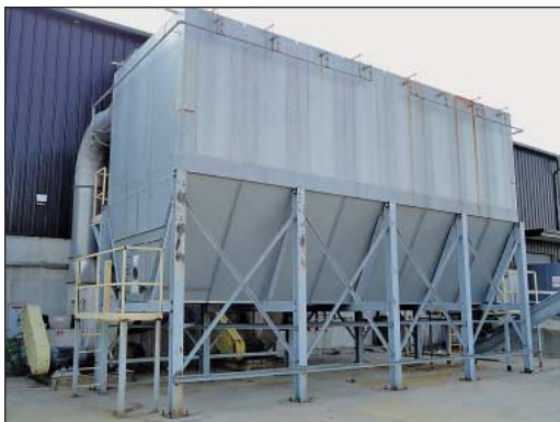
Nordfab Type NFK-6HW/2BL Bag Type Central Dust Collector
