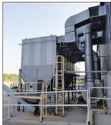
Nordfab Type NFK-6HW/2BL Bag Type Central Dust Collector
