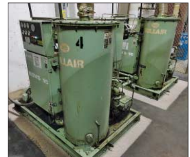
(2) Sullair Model RSV516-50A-AC Rotary Vacuum Pumps
