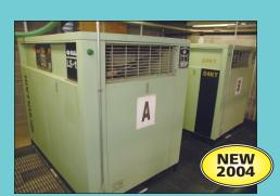
50 HP Sullair Model V-120-50 LA Rotary Screw Cabinet Enclosed Air Compressor
