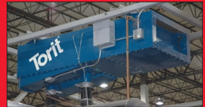
Torit Model Trunk 2000 Ceiling Hung Fume Collector
