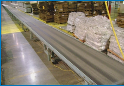
Large Quantity Various Style Conveyor - Likely To Be Sold For Scrap
