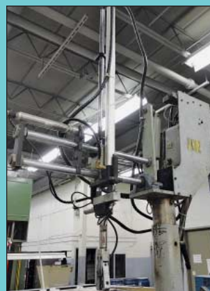
Close Up View Numerous Sprue Picker Robots
