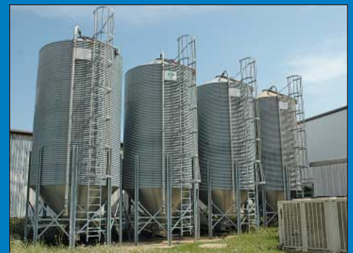
(4) 12' Dia. X 20' High IMCS Corrugated Steel Bolt Together Storage Silos
