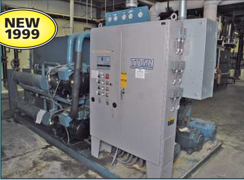
Advantage Model T1-100W-43SRX Central Water Chiller
